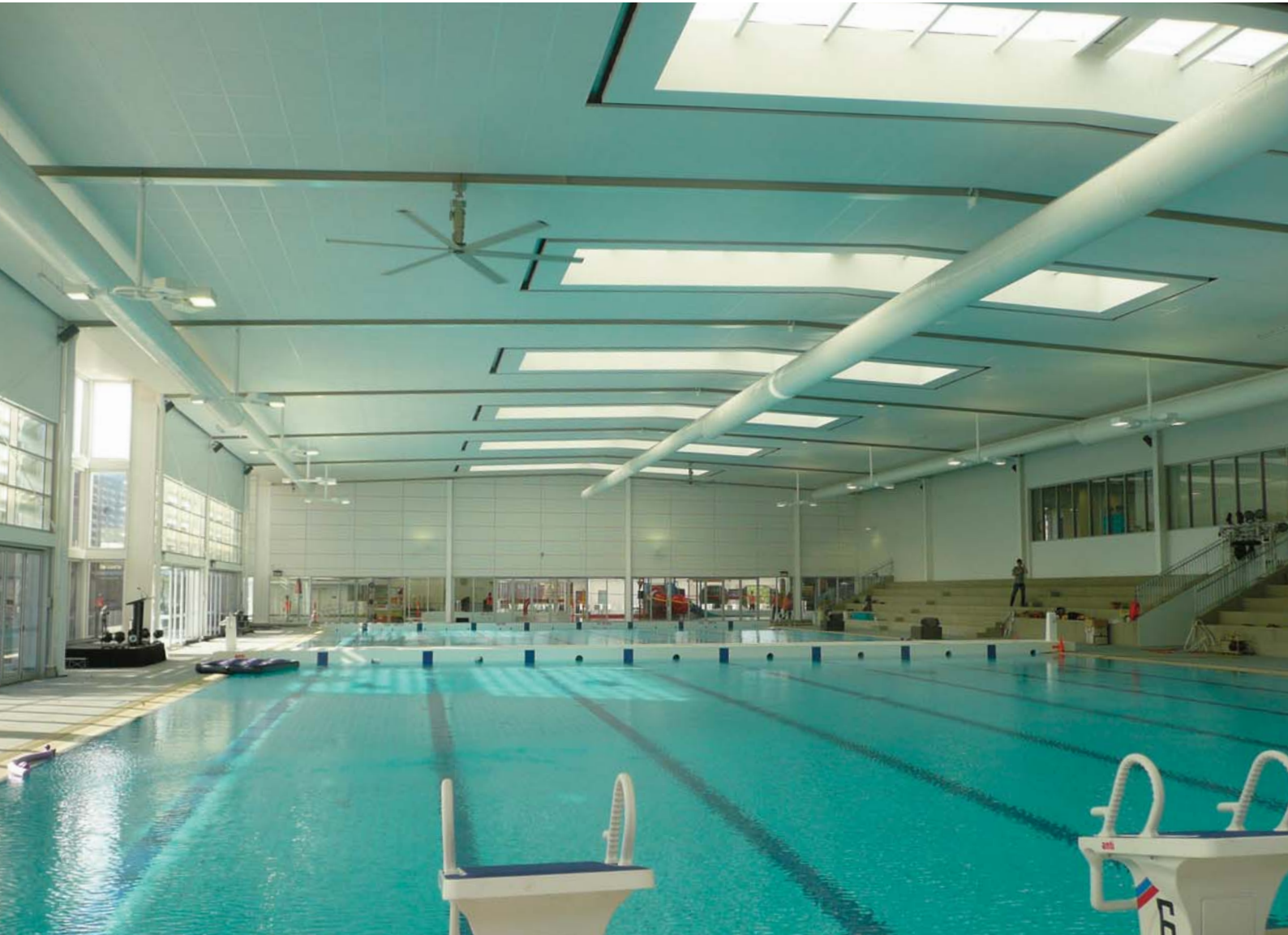
FINE FISSURED Ceramaguard with 24mm aluminium Exposed Tee grid
